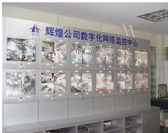
厂区全程数字化监控系统 Whole-course digital monitoring system of the plant area
