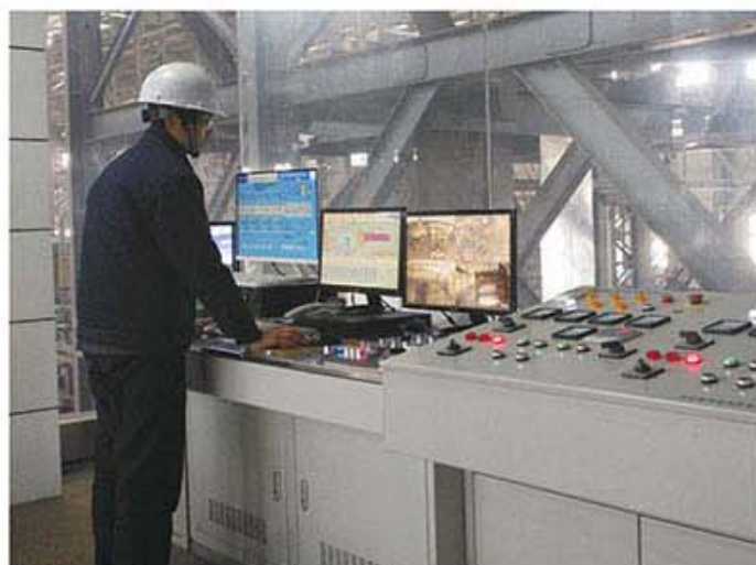
镀锌自动化操作系统 Automated operating system of galvanized producing line
